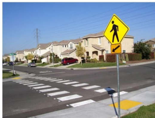
Figure 32: A triple-four crosswalk pattern. This pattern is highly-visible, has a center channel that is less slippery, and has bars spaced to reduce maintenance costs
